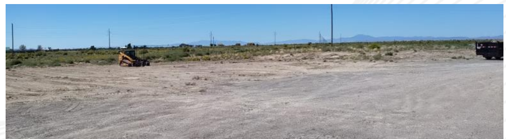
Clearing and leveling plant site
