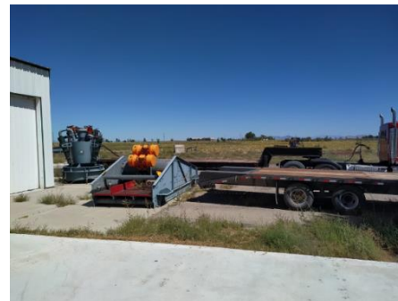
Assembling plant components
